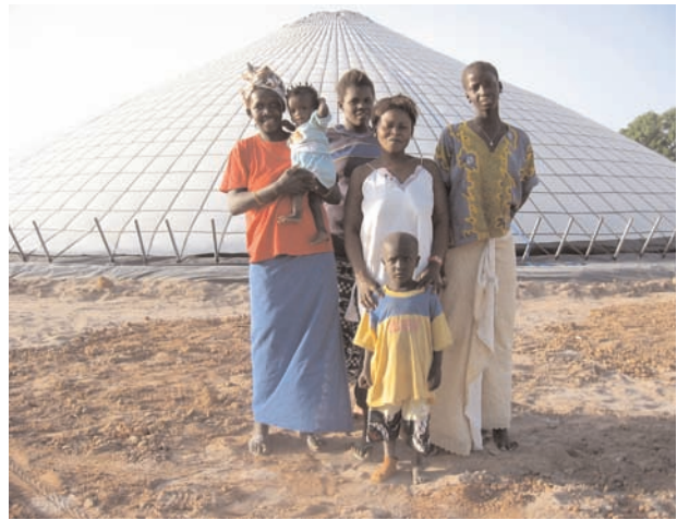
WaterPyramids are structures, placed over salty and/or contaminated bodies of water, which heat up in the sun. The water evaporates and condenses into water pure enough to be used for IV solutions; so pure, that minerals must be added for use in irrigation to ensure nutrient-rich crops. Image: Martijn Nitzsche, Aqua- Aero WaterSystems BV, Sibanor, The Gambia
