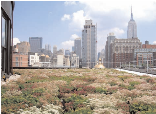
Rooftop gardens cool buildings, beautify cities and reduce the urban heat island effect. Image: Cook + Fox Architects LLP
